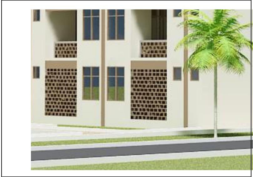
Figure 8: Concrete perforated elements on external walls
