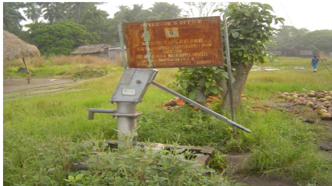
Plate 1: Abandoned Borehole Fitted with Hand Pump at Siriwon
