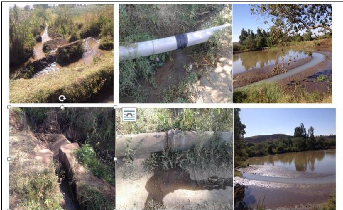
Figure 10. Irrigation water conveyance systems damaged canals (left) broken PVC (middle) and pond filled with sediments (right) (Source: own picture 2017)
